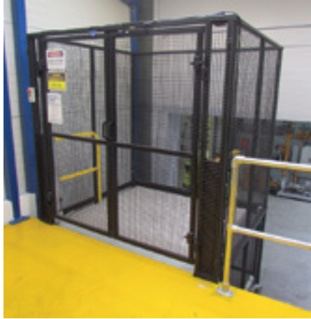
Loading bay level
