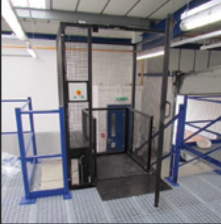
Self-supporting mesh shaft
