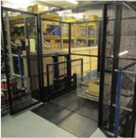
Open cage at mezzanine level
